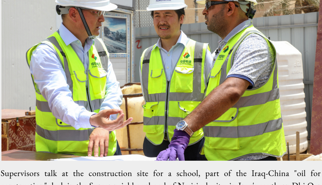
Supervisors talk at the construction site for a school, part of the Iraq-China "oil for construction" deal, in the Sumer neighbourhood of Nasiriyah city, in Iraq's southern Dhi Qar province, on July 20, 2022. China has gained a major foothold in oil-rich Iraq, shaking up Western domination in fields from energy to construction, even as some warn infrastructure projects could leave Baghdad in debt. Photo: Asaad Niazi / AFP
