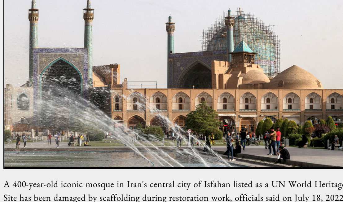
A 400-year-old iconic mosque in Iran's central city of Isfahan listed as a UN World Heritage Site has been damaged by scaffolding during restoration work, officials said on July 18, 2022. Photo: ATTA KENARE / AFP
