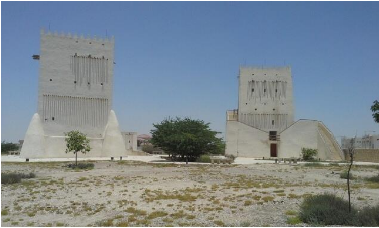
Figure 3. Al Barzan towers, used as a museum for visitors. Source: Author.
