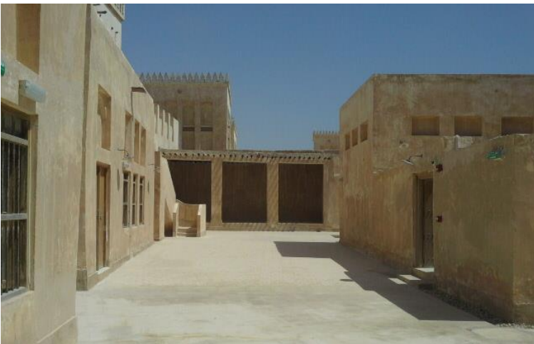
Figure 1. Al Wakrah Souq, the completed reconstruction works. Source: Author.
